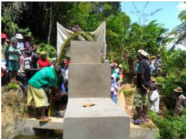
Ouvrage hydroagricole Ilamba
