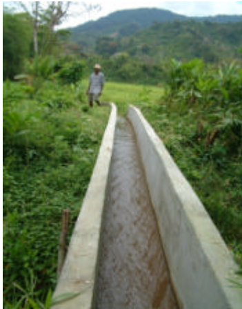
Pont canal Ankobahoba
