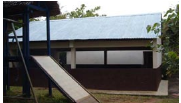
Shiny new tin roof on Education Centre.
