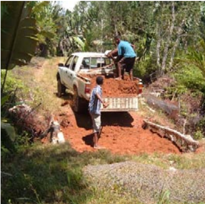
Replacing the bridges.
