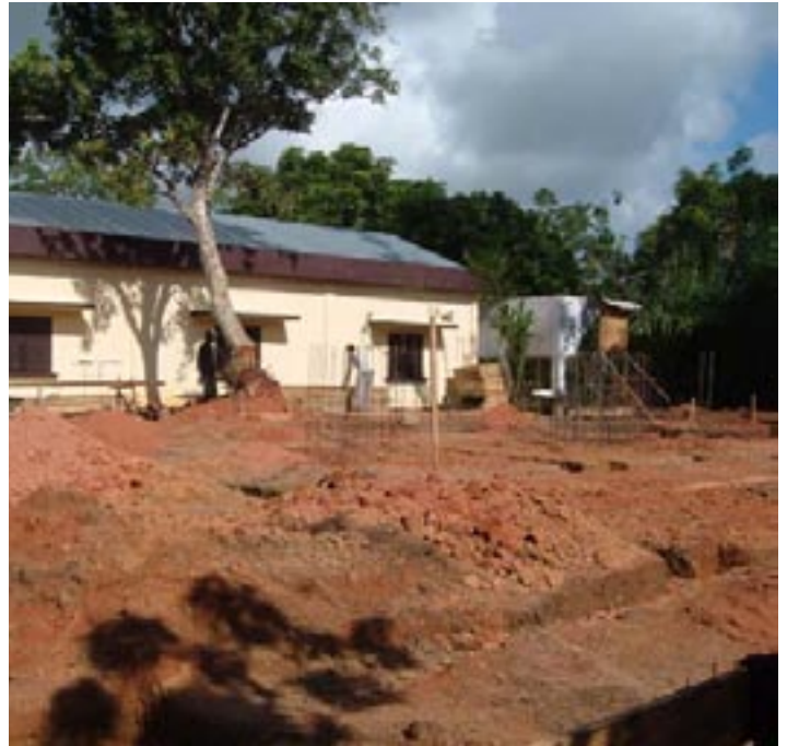
Construction is underway once more at Ivoloïna.
